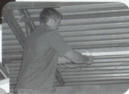
Shawn Kuhnert works on installing a new light fixture.
