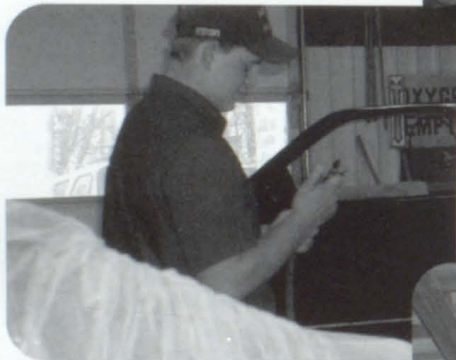
Luke Lednicky wires a light fixture.
