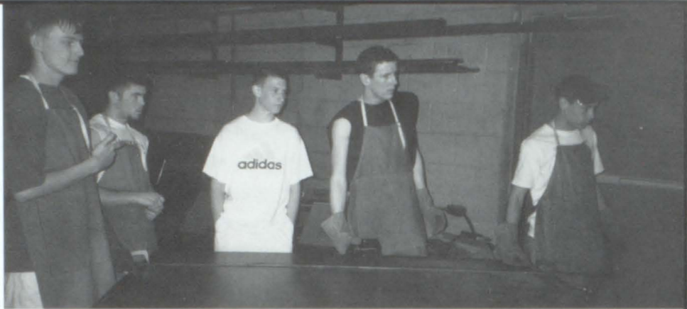
Jeff Jewell, Brett Miner, Josh Falk, and Mark Scholz prepare to cut a sheet of metal with the torch.
